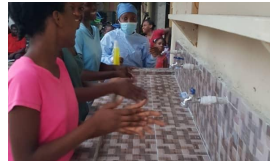
The new hand washing station.
